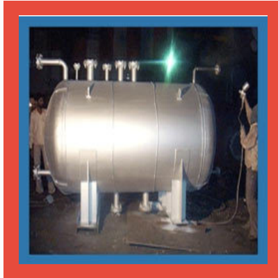
Mild Steel Fabrication Work
